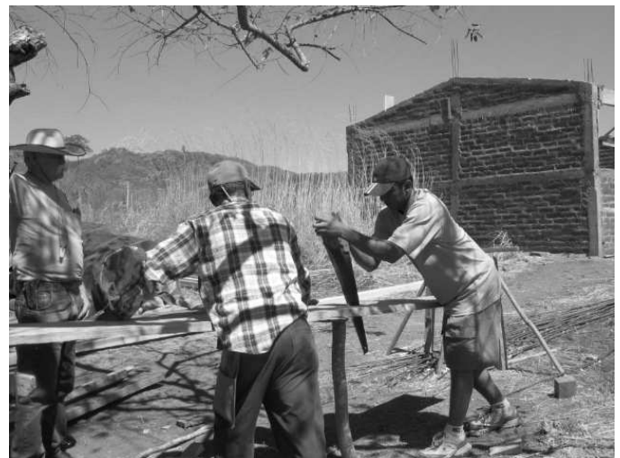
Sawing boards for the new La Poma school.
